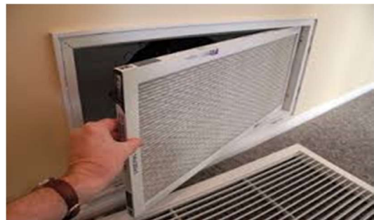
Filter in wall
